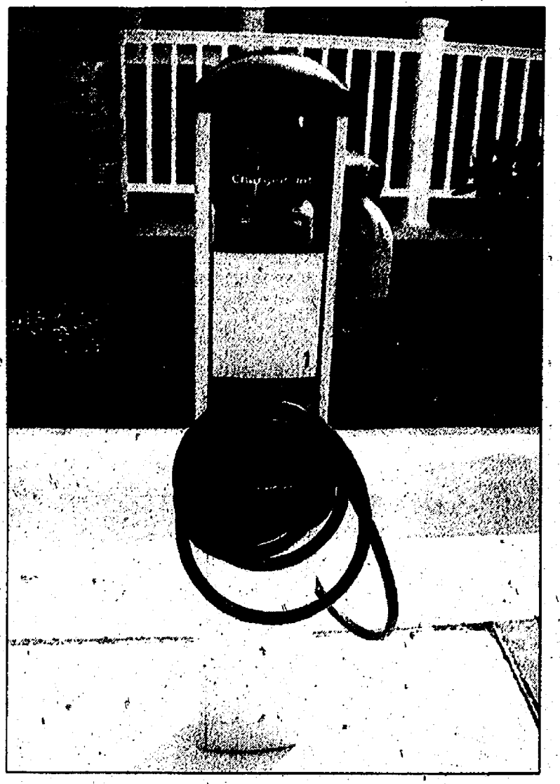
This station, which recharges electric vehicles like the Chevy Volt and the Nissan Leaf, provides a fast way for drivers to recharge. The station is provided to drivers for free.
